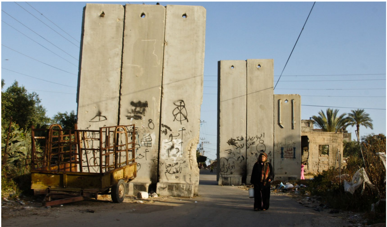
FIGURE 2.12 SALVAGED CONCRETE BARRIERS
