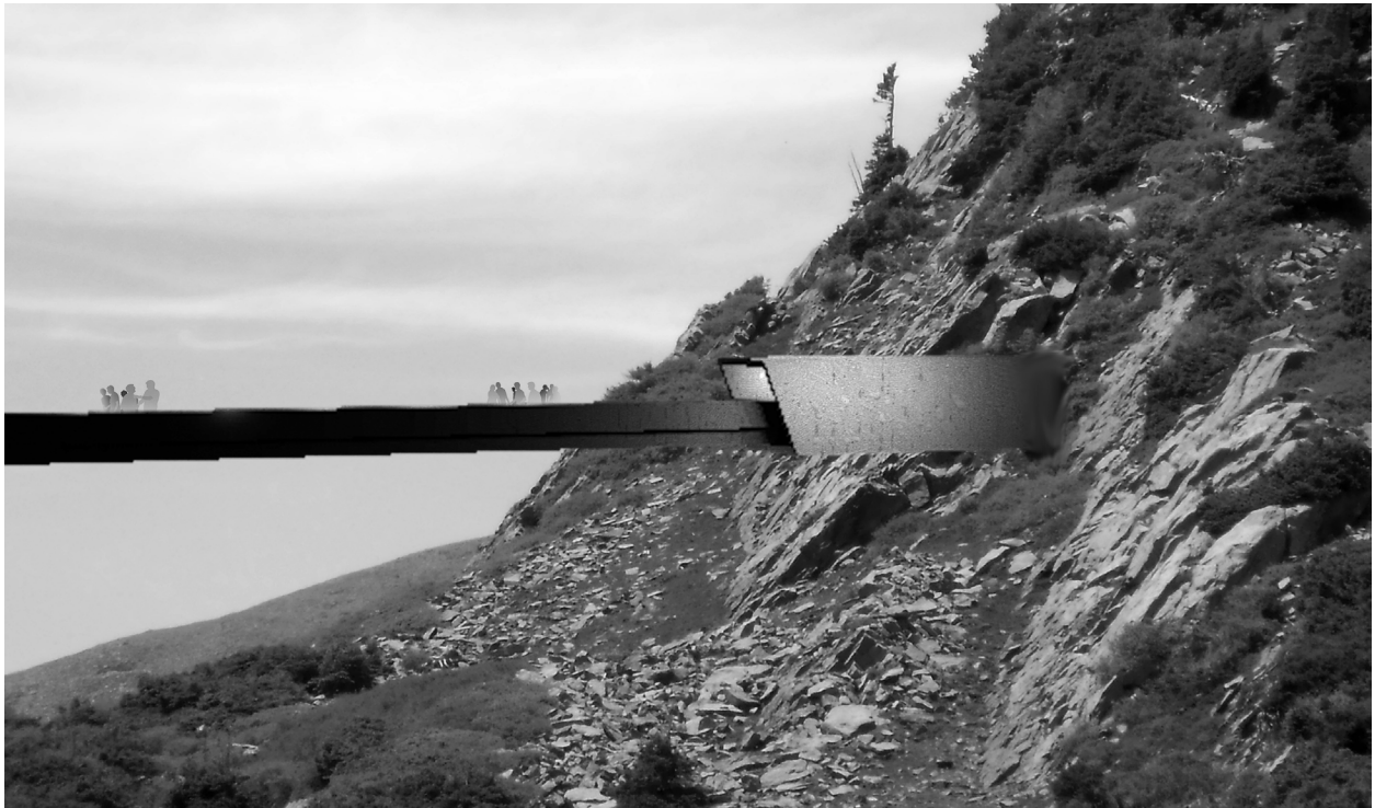
FIGURE 4.21 PUNCTURING THE MOUNTAINSIDE
