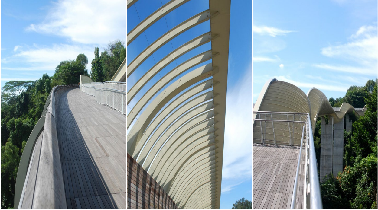
FIGURE 4.9 HENDERSON WAVES BRIDGE, ASSORTED VIEWS
